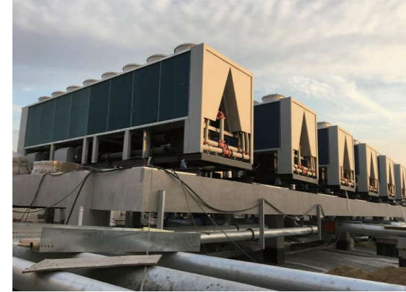
Fig.1 Installation site of the air-cooled chiller for the computer room
