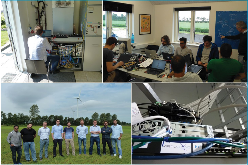
Figure 12. Field trials of VirtuWind solution at "Floe" wind park (Denmark)
